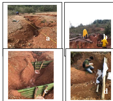
Figure 2.a-Ravine, b- Palisades construction, c-Built Palisade, d- Palisade Monitoring.
